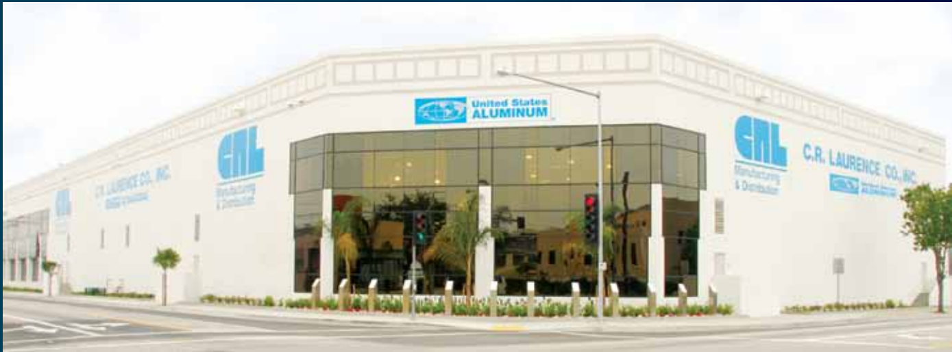
The New U.S. Aluminum Facility in Los Angeles, California
